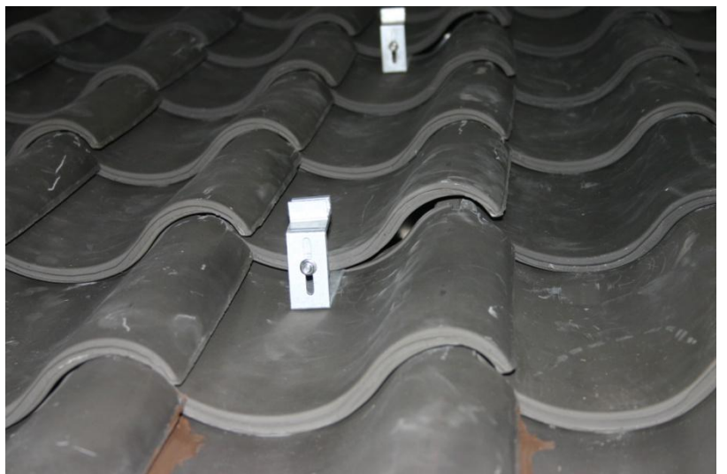
Photo 12 Detail of test specimen 3B, tile not grinded.
